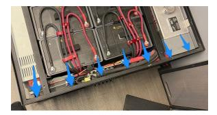
1.5. Remove twelve screws holding panel to wall
